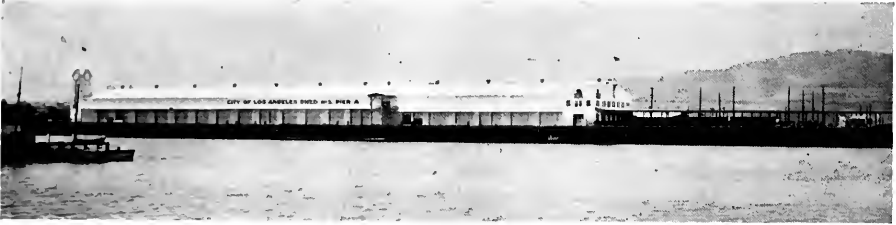
Municipal shed No. 3, Pier A, and a portion of the wharf erected by the City of Los Angeles for the use of the Pacific S.S. Co. The shed is 622 feet long and 100 feet wide and is equipped with passenger facilities as well as for freight. The entire wharf is 1427 feet long. An umbrella shed, 290 by 60 feet, has just been built at the other end of the wharf.
